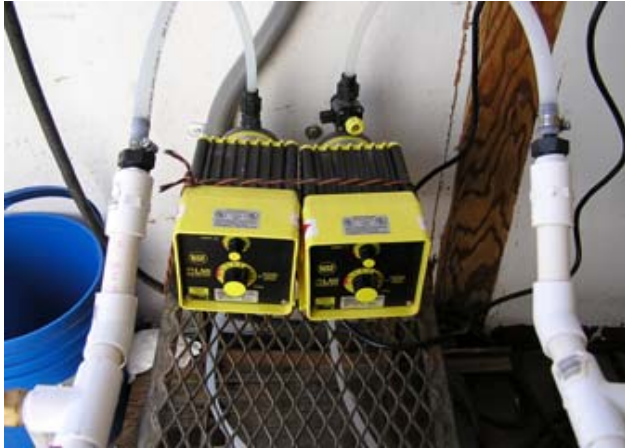
Independently meter both solutions from the tanks...
