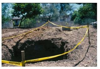
Four steel fuel storage tanks (2 diesel, 1 gasoline and 1 bunker oil) were excavated from various locations on a residential property. Soil samples were collected and analyzed for total petroleum hydrocarbons (TPH) which indicated soil contamination was present (the highest TPH concentration was 8,100 mg/kg).
