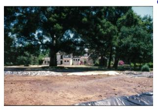
The County Health Services Agency requested that the contaminated soil be disposed at an appropriate facility. BioWorld teamed up with an engineering company and proposed bioremediation as a viable option.
