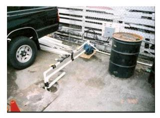
Underground storage tanks were removed from an old service station in the mid 1990's. Gasoline had leaked out of the tanks and contaminated the shallow groundwater. An engineering firm was hired to begin the cleanup and 6 monitoring wells were installed. After 7 years of monitoring, there were no changes in the analytical tests and the firm was released. BioWorld teamed up with a progressive and innovative engineering firm determined to clean up the groundwater.
