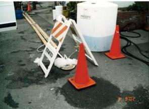
BioWorld Bioremediation Enhancer and Hydrocarbon Digesting Microbes were added several times down the monitoring wells. Within 5 days, 8 inches of free floating product had been degraded. Treatment continued for 3 months with a 90% reduction in dissolved phase gasoline constituents verified.
