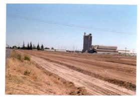
Old wooden fuel storage tanks were excavated 6,000 cubic yards of contaminated soil was spread over a 4 acre area in treatment parcels 1 foot deep.
